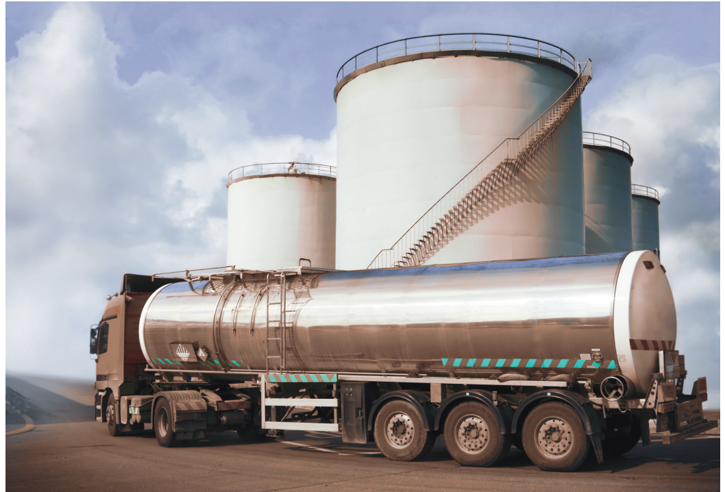
Remote tank-level monitoring systems improve efficiency, logistics management and inventory control in the distribution of petroleum and chemical products stored in tanks.
